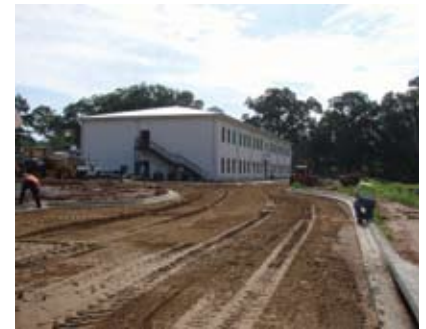
Imagine School at Evening Rose under construction.
